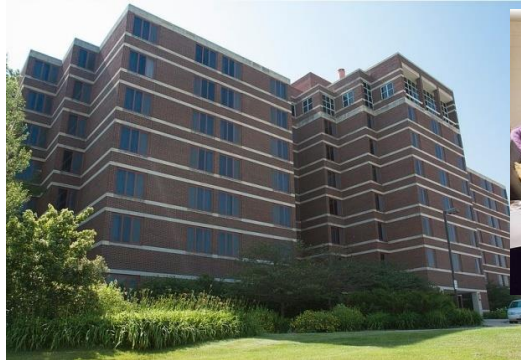
Farwell Hall on Luther College campus.
